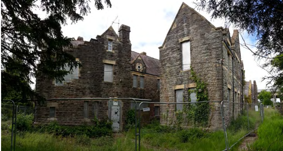
Figure 11 - 1896 'baronial' entrance range
